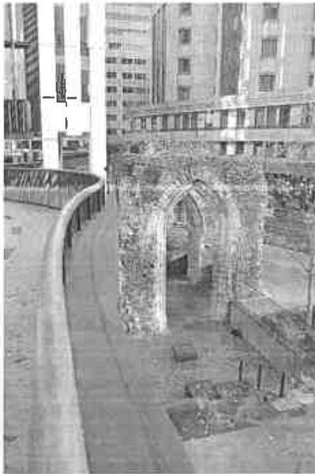
Figure 1 The 14th-century tower of Elsing Spital viewed from the walkway in the London Wall development; explanatory plaques will be fixed to the railing of the walkway and at ground level on London Wall
